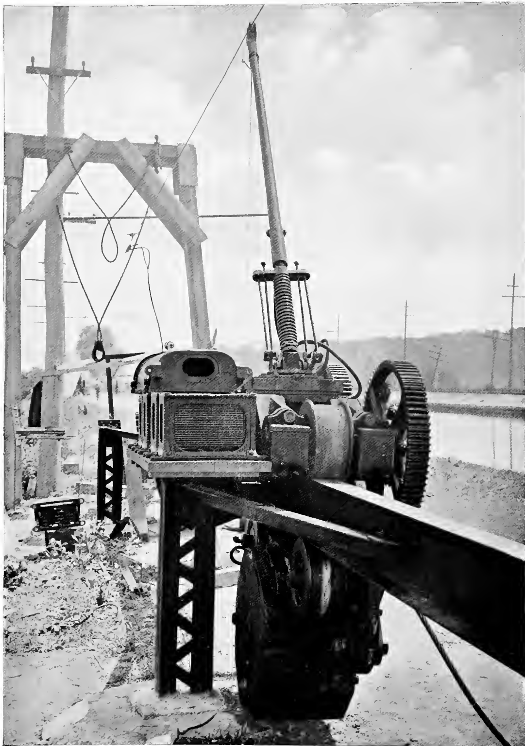
ELECTRIC CANAL TRACTOR (WOOD SYSTEM)
